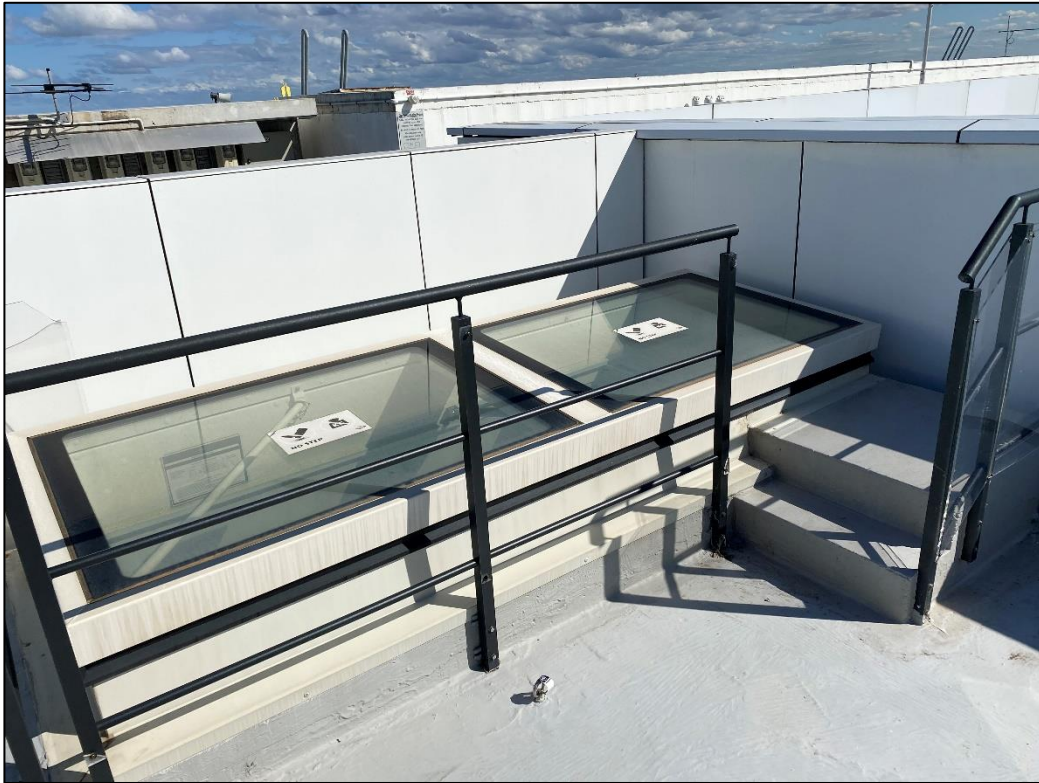
Figure 6: Glass roof access hatch on the roof top
